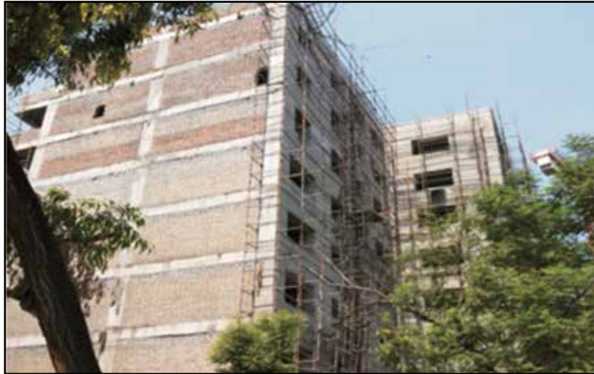
Construction of 8+1 PG Building
